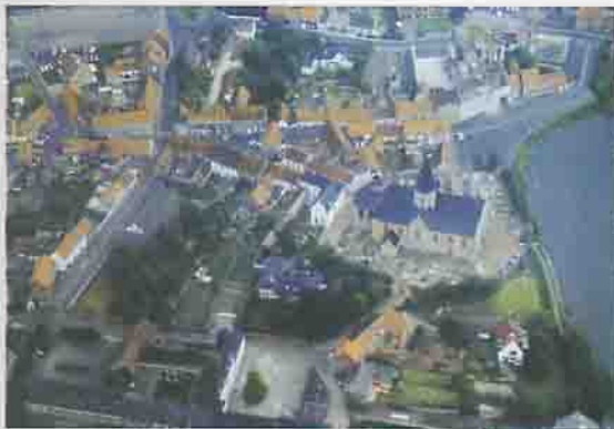
Vista del estado previo | View of previous condition
